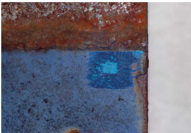
Figure 3 Detail of One for Bristol . A scratch test revealed the original paint finish underneath.
