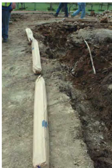
Figure 10a Installing a cathodic protection system on Rumi . Bags of magnesium powder are shown before being placed in the trench around the sculpture.
