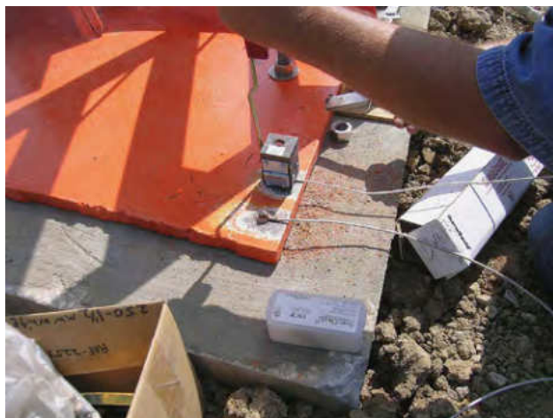
Figure 11a A thermite explosive charge is used to produce an extremely high temperature that bonds the cables instantly to the sculpture's clean metal surface.
