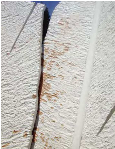
Figure 6 Areas of touch-up on a feather of one of the Shuttlecocks . Over time the touch-up paint could not be matted down sufficiently to match, with aesthetically displeasing results.
