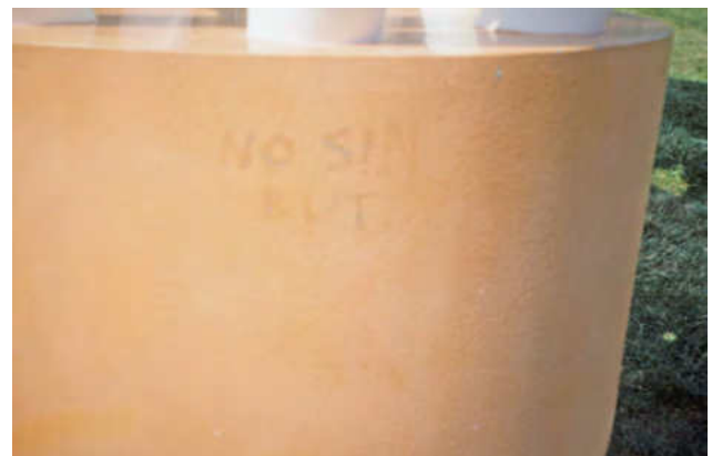
Figure 5 Chalked, faded orange paint and graffiti on one of the Shuttlecock balls about three years after installation. By this point, periodic polishing and buffing was no longer effective in remediating the damage.
