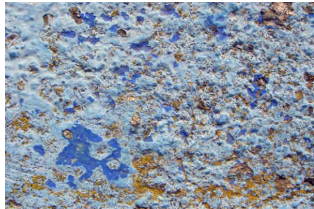
Figure 9 Detail of Energia Mediterranea , showing clear evidence of previous, darker paint layers beneath the existing faded blue, alongside deterioration products of the paint and concrete. Photo: Tom Learner.
