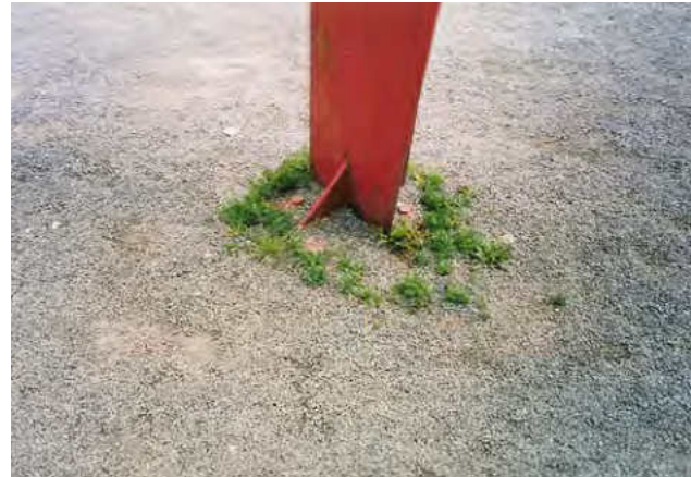
Figure 8 Corrosion damage is evident on the feet of the sculpture, caused by gravel with grass growing over the base plates. © 2014 Calder Foundation, New York / Artists Rights Society (ARS), New York. © ZMK, Hannover 2003.
