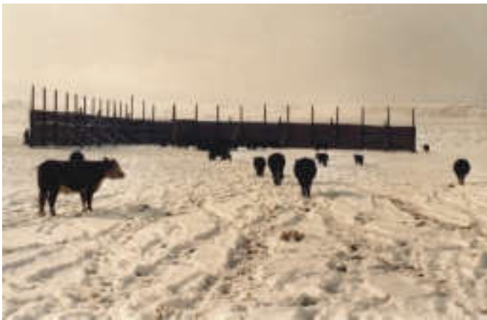
This windbreak structure located at Miracle Mile in Carbon County, Wyoming, provides protection from cold winds, raising the effective temperature of cattle behind the windbreak.
