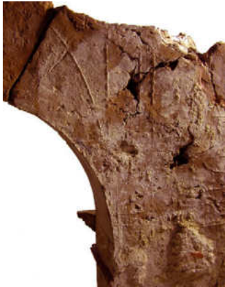
Figure 4. Ranking light detail of the back of the arch with incise marks of the wooden board. © IMC-DGPC
