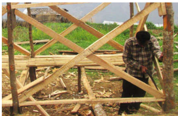
Fig. No. 2.4.3.1 Constructing earthquake resistant goat shed using cross beam
