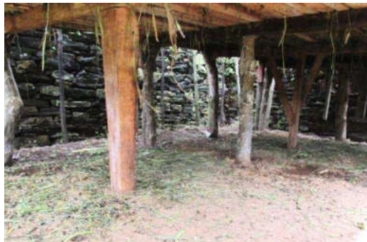
Fig. No. 2.4.4.1 Shed in good condition – clean and dry
