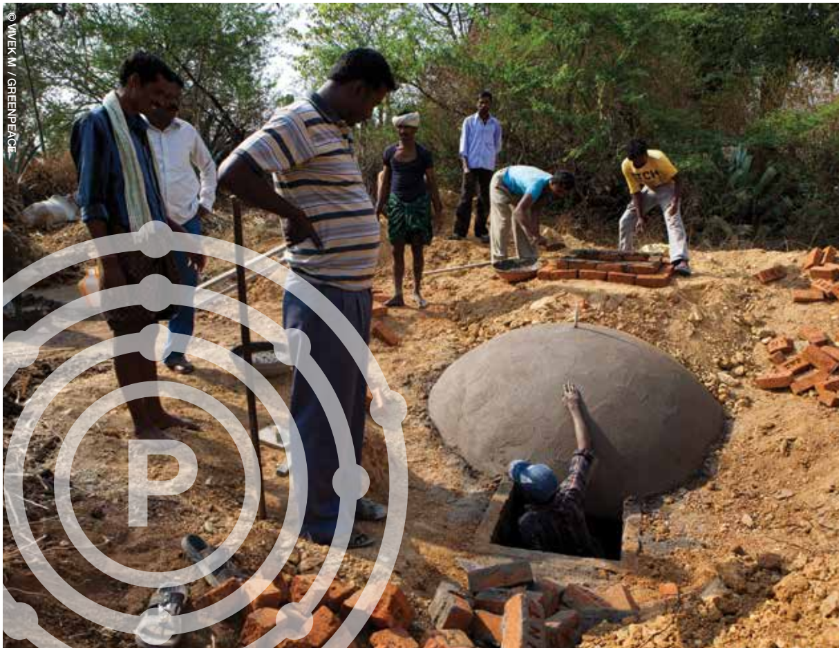
Image Workers building a new biogas unit in Kammavaripalli, Bagepalli taluk, India.
