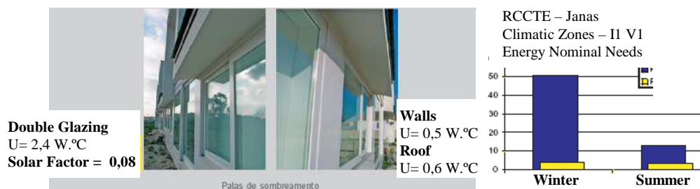
Figure 10. Thermal conductivity coefficient of walls and glazing.
