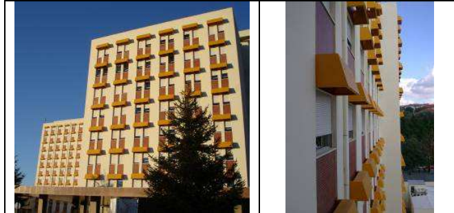
Figure 6. Glazing / Shades Solar Control.
