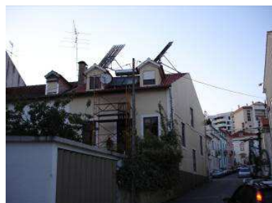
Figure 5. Wrong implementation of solar systems.
