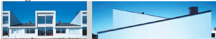
Figure 7. Photos from the South and West facade.
