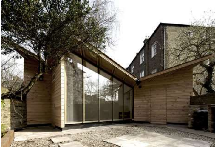
Fig. 52 The saw-toothed frontelevation which maximises natural daylight and passive solar heating to the interior.
