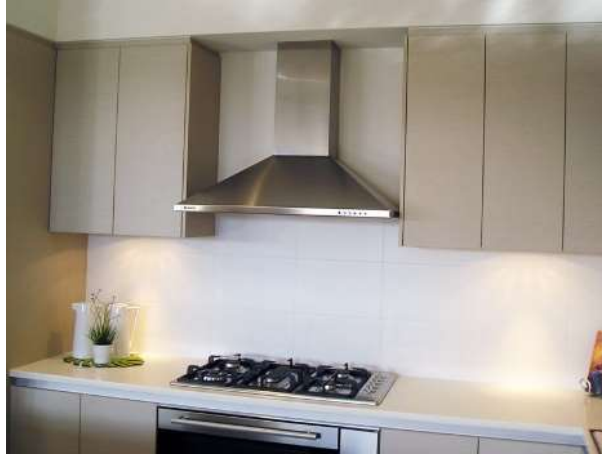
Fig. 77 Installing a rangehood in a kitchen sucks in the moisture from cooking
