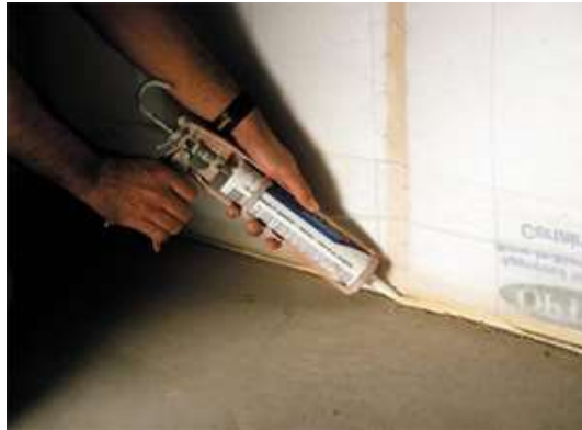
Fig. 55 Caulking the cracks
