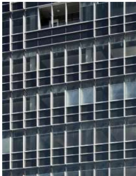
Fig. 142 Facade of the Environmental Protection Agency (Green Team 2013)
