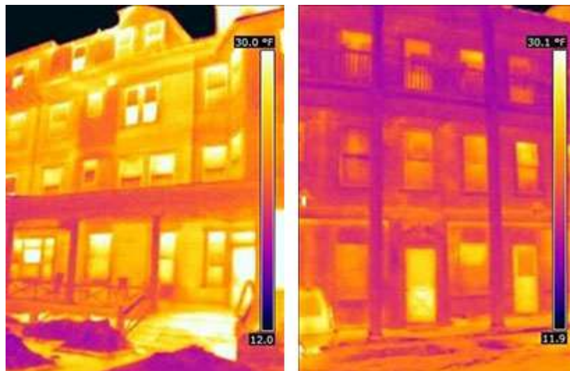
Fig. 97 Thermal photo of a building
