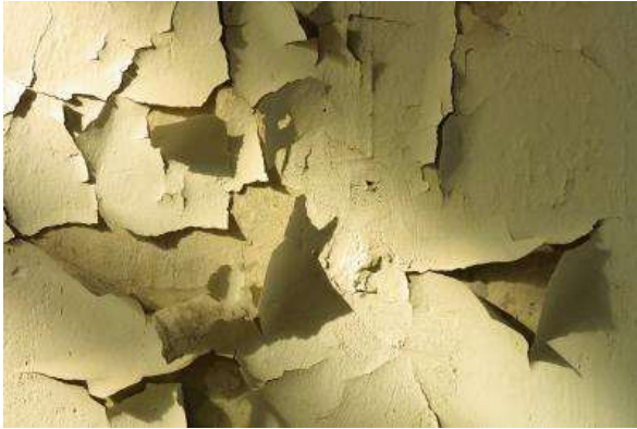
Fig. 74 Peeling paint
