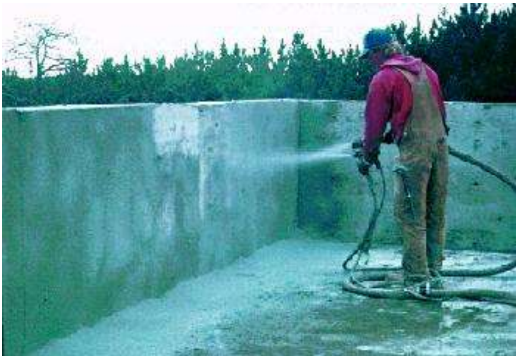
Fig. 72 Bentonite waterproofing being sprayed on a home recently completed in Missouri
