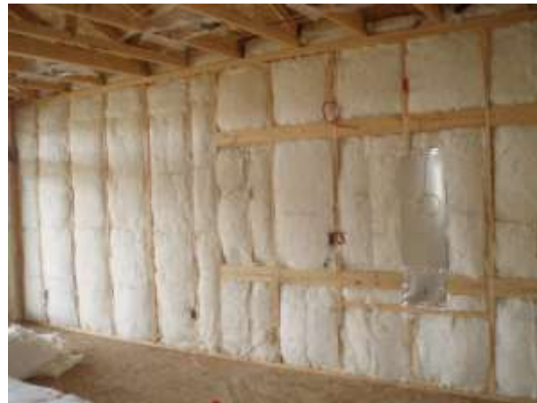
Fig. 78 Higher temperatures usually mean less humidity – installing an insulation in wall heightens the temperature and makes humidity lower
