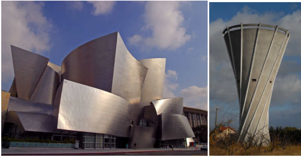
Figure 10: Two usages of particular curved surfaces. Left: The Los Angeles Walt Disney Concert Hall with a stainless steel façade, piece-wise developable, image by J. Sullivan (2004), courtesy of PDPPhoto.org. Right: Water tower in La-Roche-de-Glun (France), with a one-sheet hyperboloid ruled surface; image by A. Rambaud (2007), with permission
