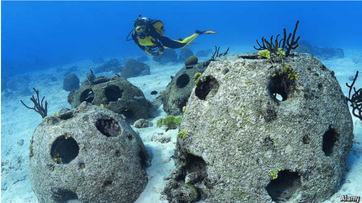
Figure 21.12. Artificial reefs created based on the mold/process promoted by the Reef Ball foundation. The holes in the balls are to facilitate the movement of small fish and invertebrates in and out of the Reef Ball.
