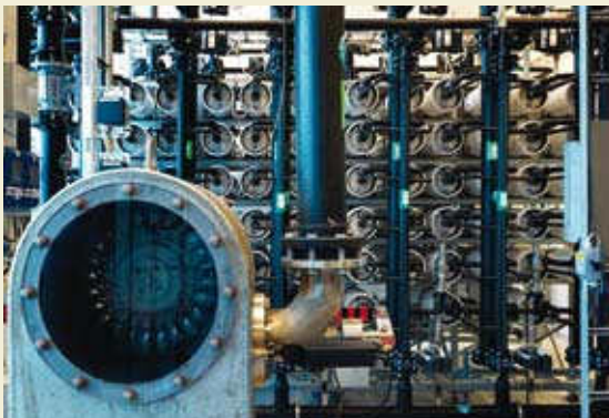
7.12 d > The world's first osmotic power plant on the Oslo Fjord in Norway derives energy from the differences in salt concentration between saltwater and freshwater. A thin membrane separates the water masses, building up pressure which drives a turbine.
