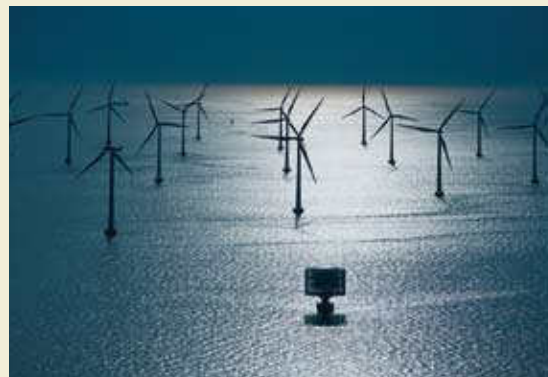
7.12 e > Offshore wind turbines produce electricity in many places around the world. One of the largest offshore wind farms, consisting of 48 turbines, is located in the Baltic Sea between Denmark and Sweden. A transformer station has been constructed here to feed power into the Swedish grid.
