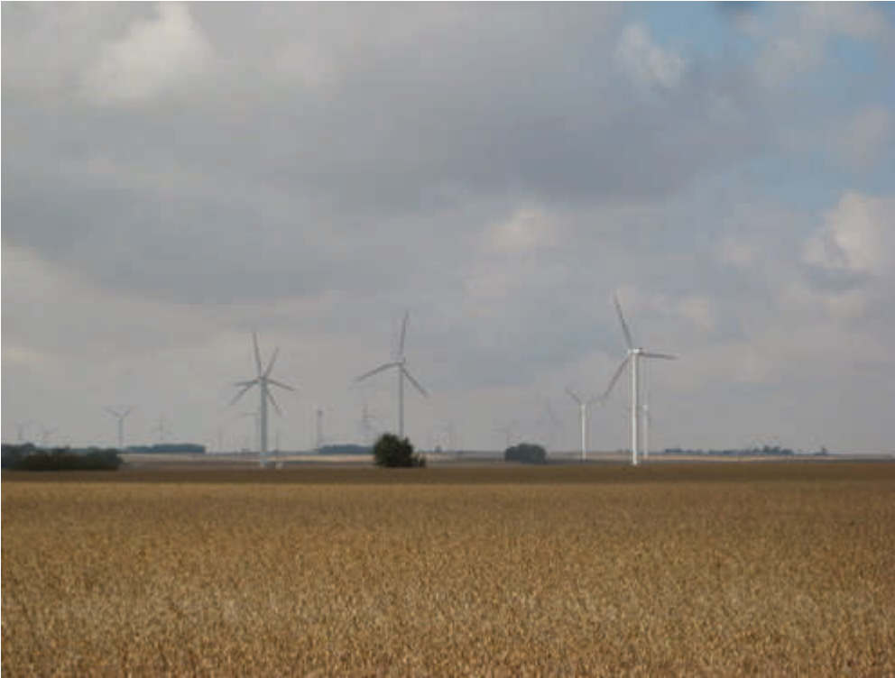
Figure 5. Twin Groves Wind Farm, Illinois Wind power is becoming a more popular source of energy in the United States. Source: Office of Sustainability, UIC
